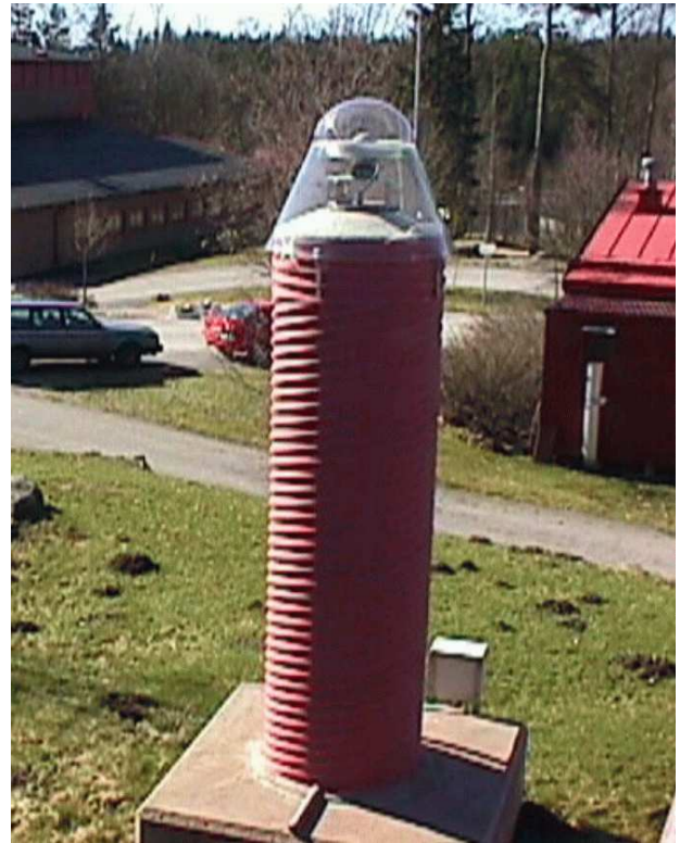
Figure 2: SWEPOS/IGS SPT0 in Borås, uses a temperature-stabilized antenna cable in a water bath.
